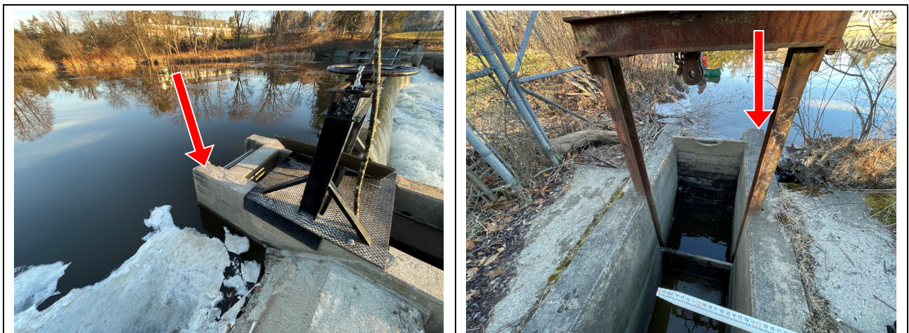
Figure 2. Locations of water surface elevation measurements for the downstream reach at Bridge Street Dam (left photo) and the upstream reach at Elm Street Dam (right photo)
